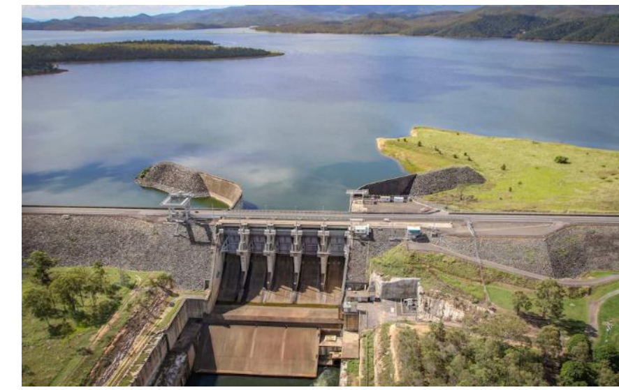
Wivenhoe Dam (1970s)
